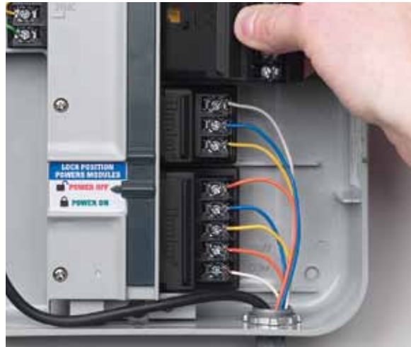
Use color-coded irrigation wire to connect the valves to the controller. You will need one wire for each valve, plus one common wire.
