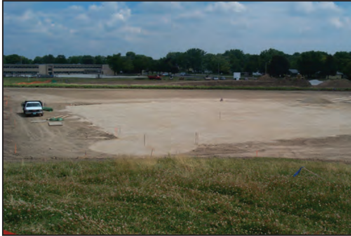
Bare soil during sports field construction - Picture courtesy of Aaron Volkening, P.E.
